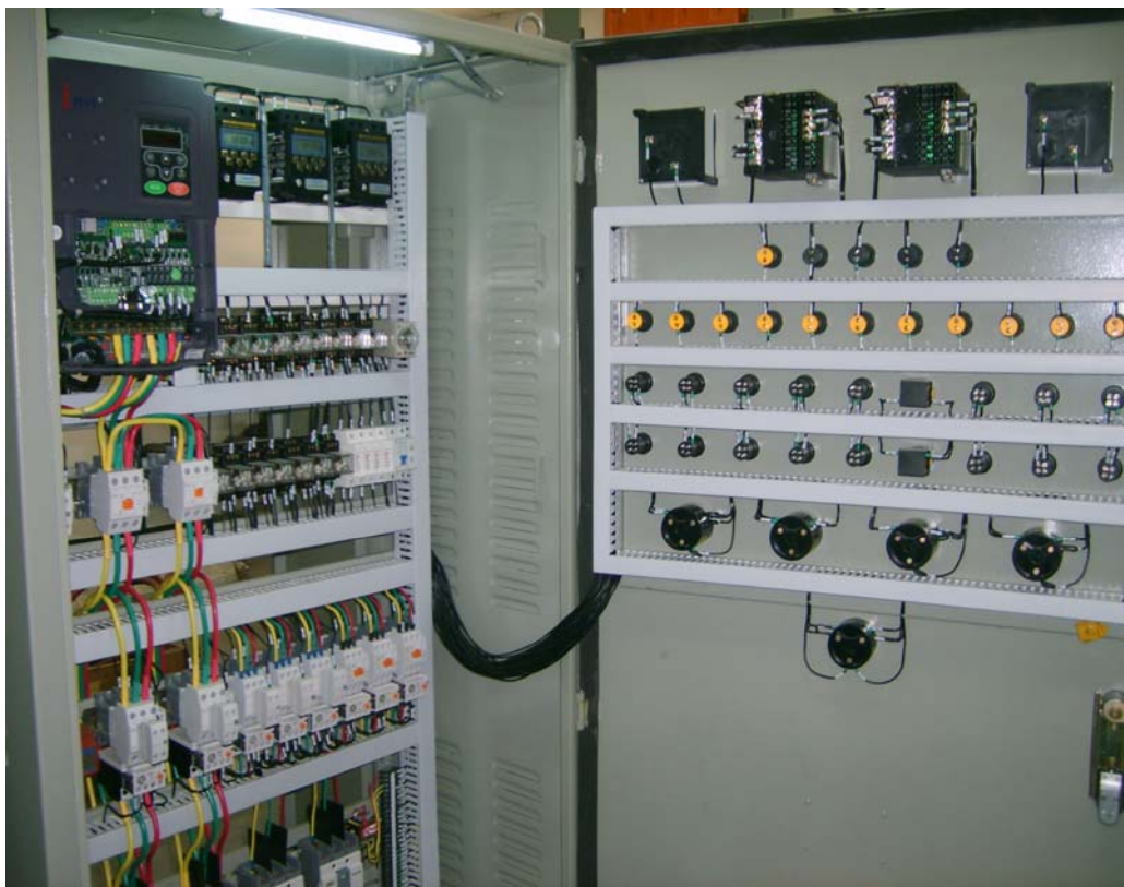
Wiring in Automatic Constant Pressure Water Supply Cabinet (2)
